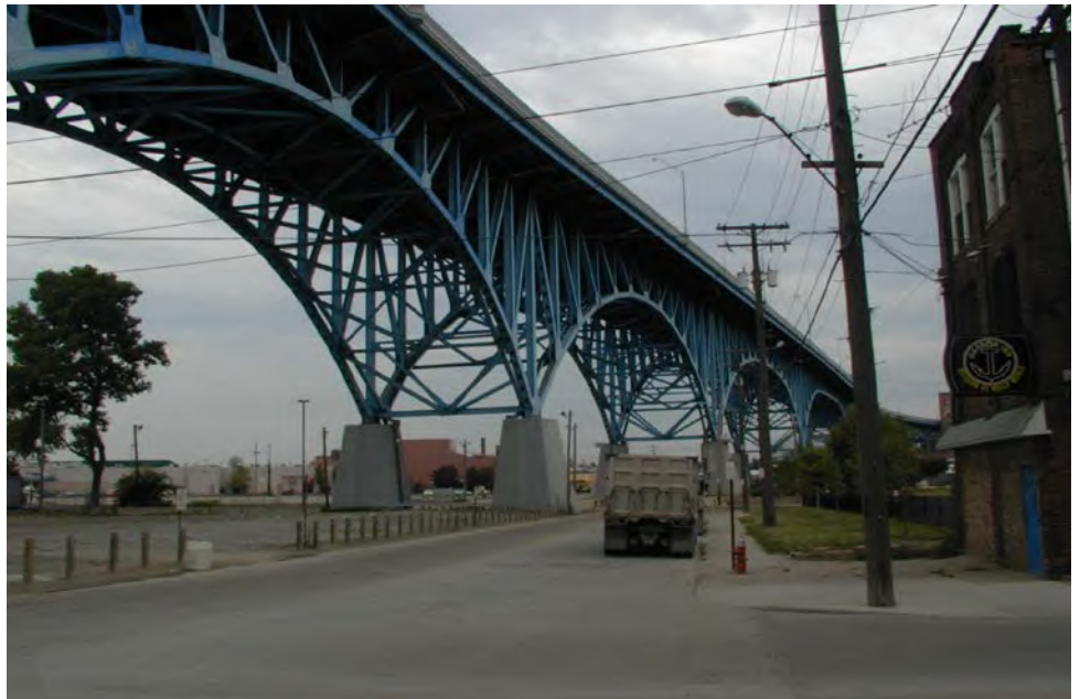
Figure 3.1.52 Deck Truss Bridge
