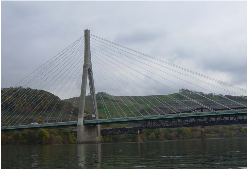
Figure 3.1.20 Cable-Supported Bridge: Cable Stayed
