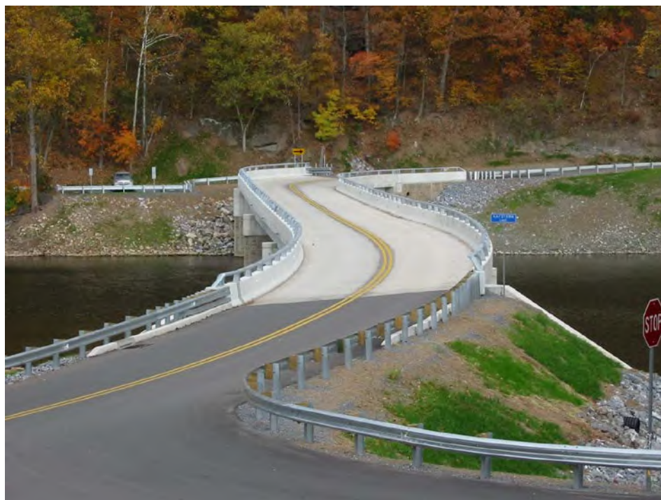
Figure 3.1.28 Bridge Deck with a Smooth Riding Surface
