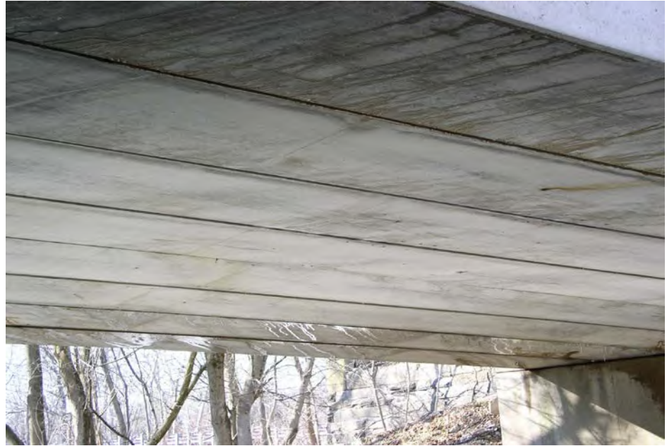
Figure 3.1.50 Adjacent Box Beam Bridge
