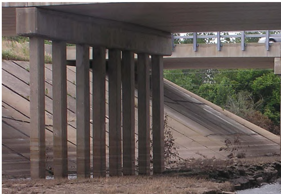
Figure 3.1.10 Concrete Pile Bent
