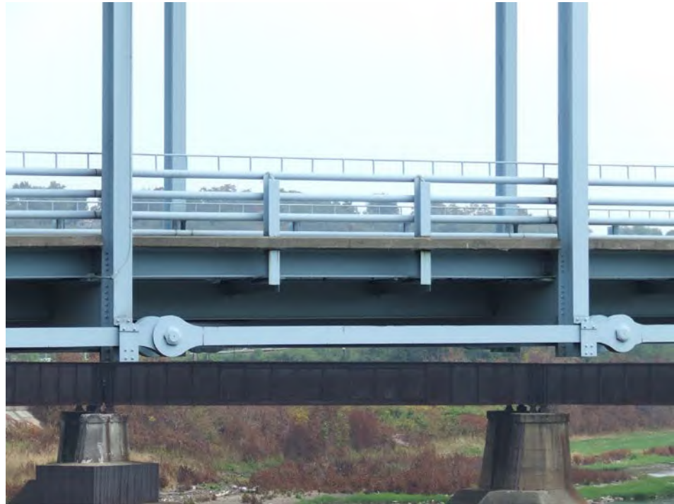
Figure 3.1.22 Pin-Connected Eyebars
