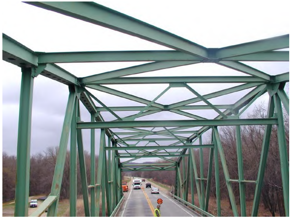
Figure 3.1.67 Top Lateral Bracing and Sway Bracing
