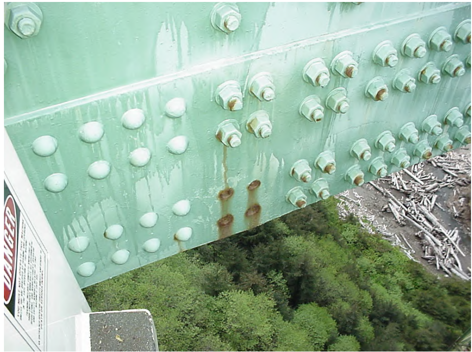
Figure 3.1.24 Shop Rivets and Field Bolts
