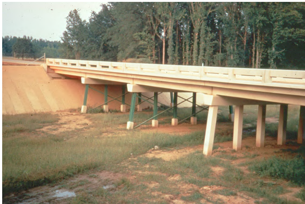
Figure 3.1.81 Pile Bent
