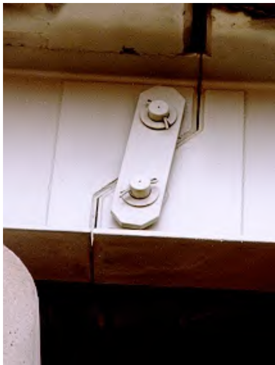
Figure 3.1.26 Pin and Hanger Assembly
