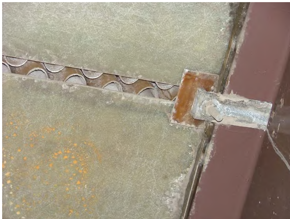
Figure 3.1.35 Fiber Reinforced Polymer (FRP) Deck
