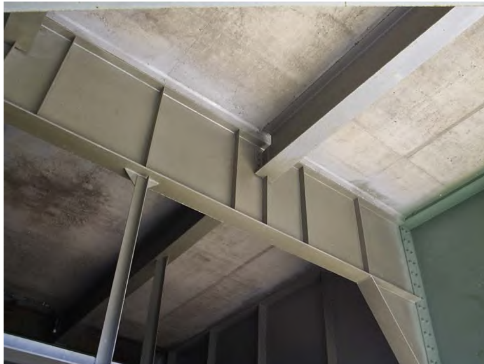
Figure 3.1.29 Underside View of a Bridge Deck
