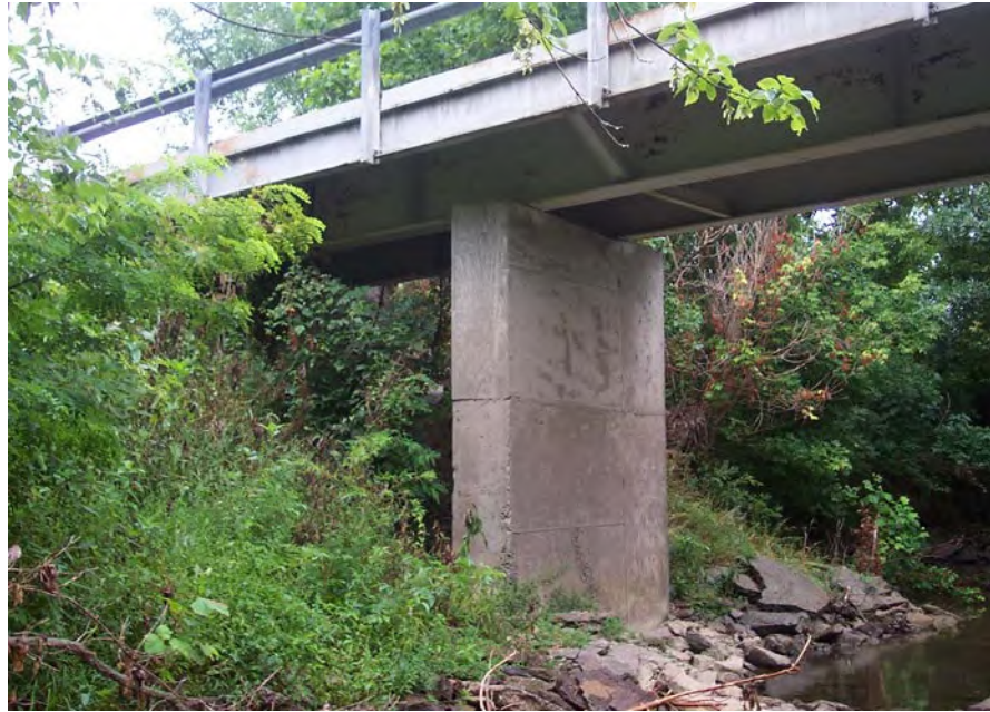
Figure 3.1.75 Solid Shaft Pier
