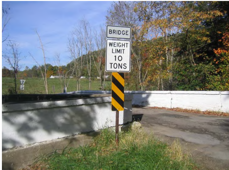
Figure 5.1.19 Bridge Weight Limit Posting
