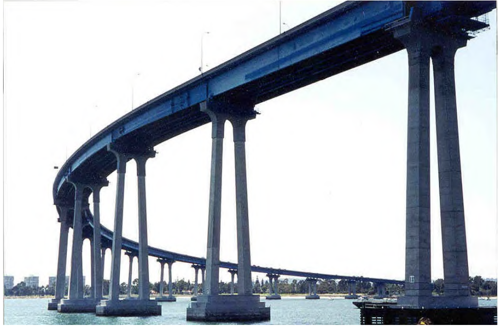
Figure 3.1.48 Curved Girder Bridge
