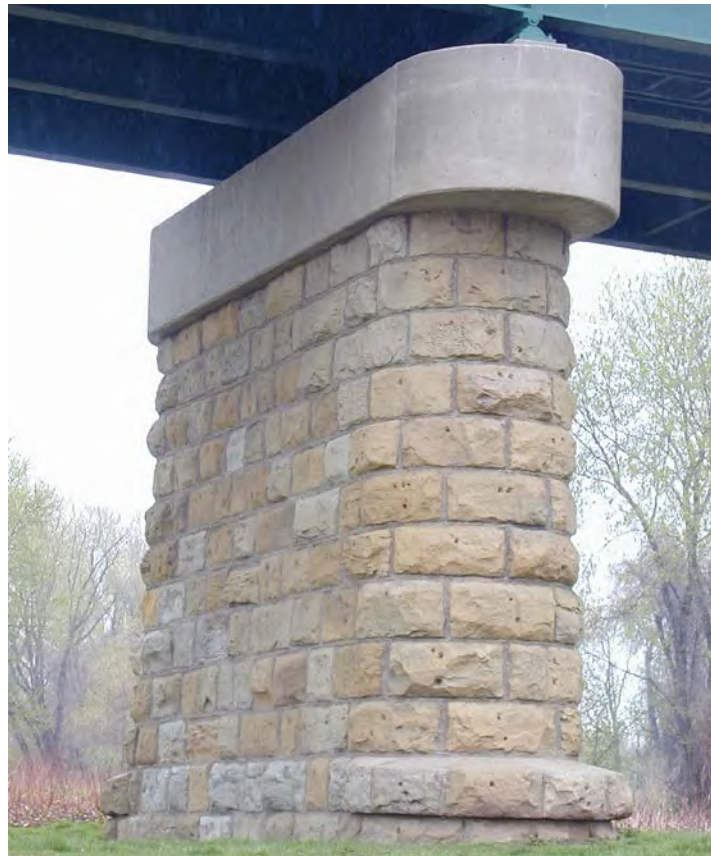
Figure 3.1.76 Solid Shaft Pier
