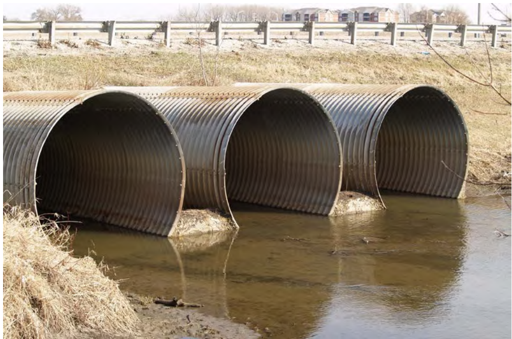
Figure 3.1.84 Flexible Culvert
