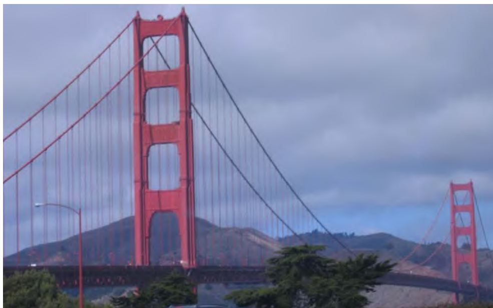
Figure 3.1.19 Cable-Supported Bridge: Suspension Cables and Hangers
