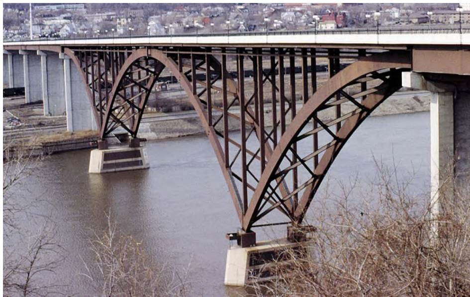
Figure 3.1.64 Main Supporting Members of Deck Arch
