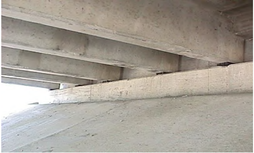
Figure 3.1.72 Stub Abutment
