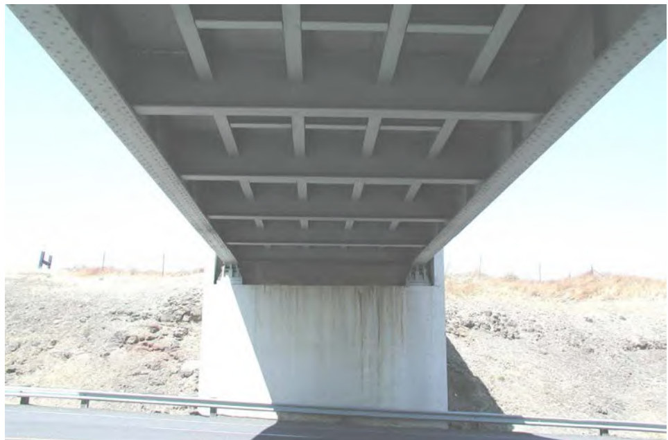
Figure 3.1.47 Girder Floorbeam Stringer Bridge
