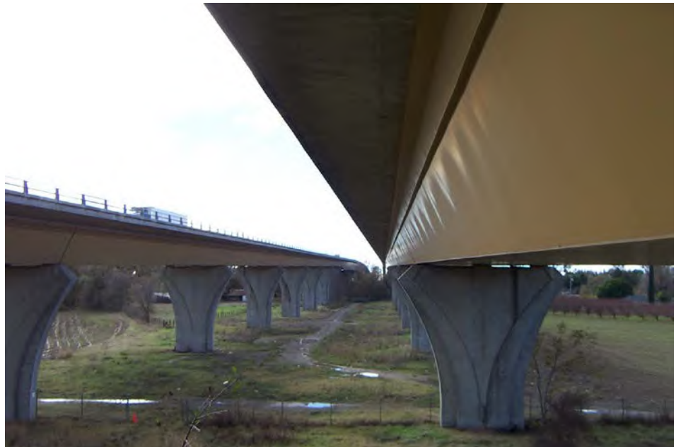
Figure 3.1.51 Box Girder Bridge
