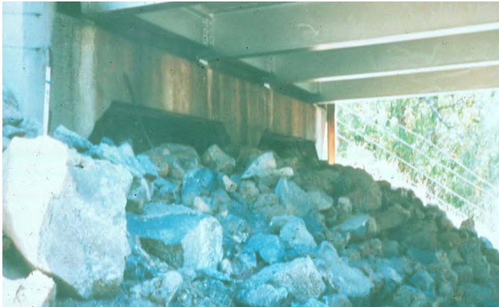
Figure 3.1.73 Spill-Through or Open Abutment
