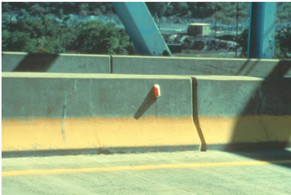
Figure 3.1.40 New Jersey Barrier
