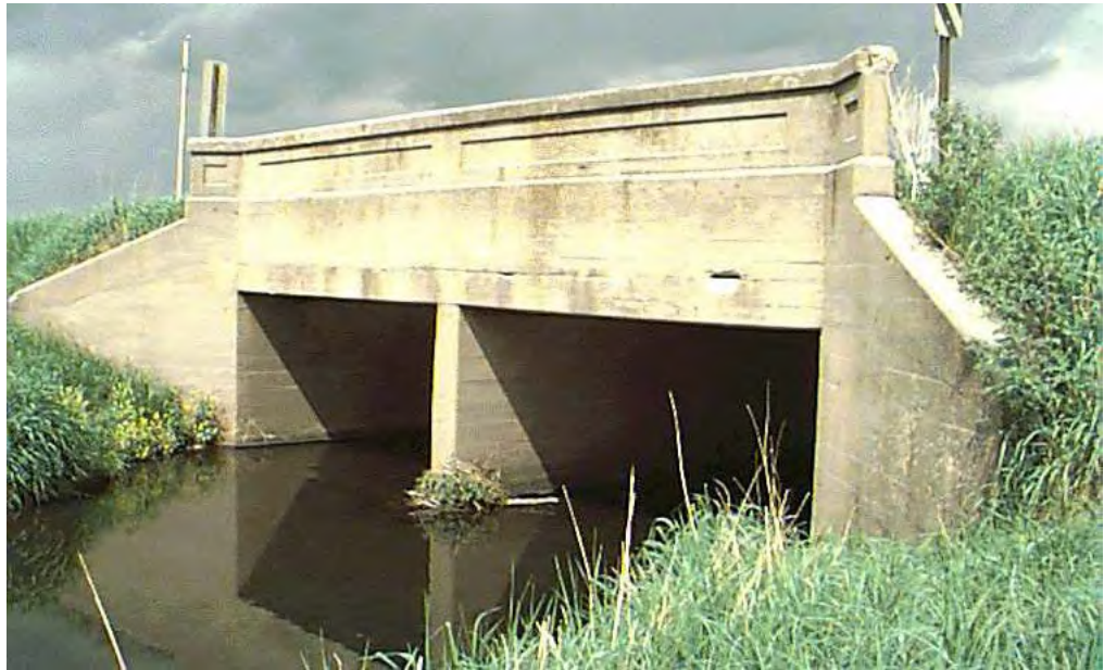
Figure 3.1.83 Rigid Culvert
