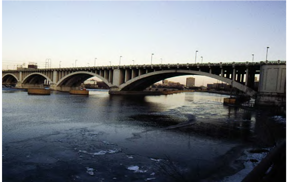
Figure 3.1.54 Deck Arch Bridge
