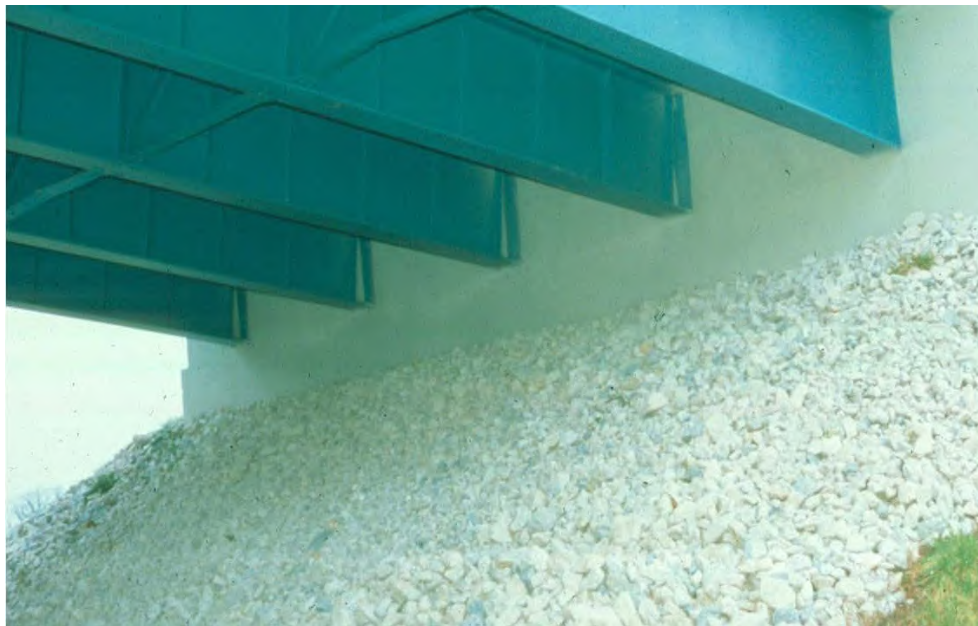
Figure 3.1.74 Integral Abutment
