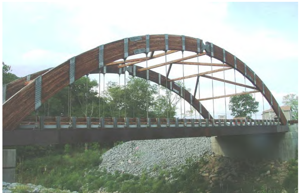
Figure 3.1.55 Through Arch Bridge
