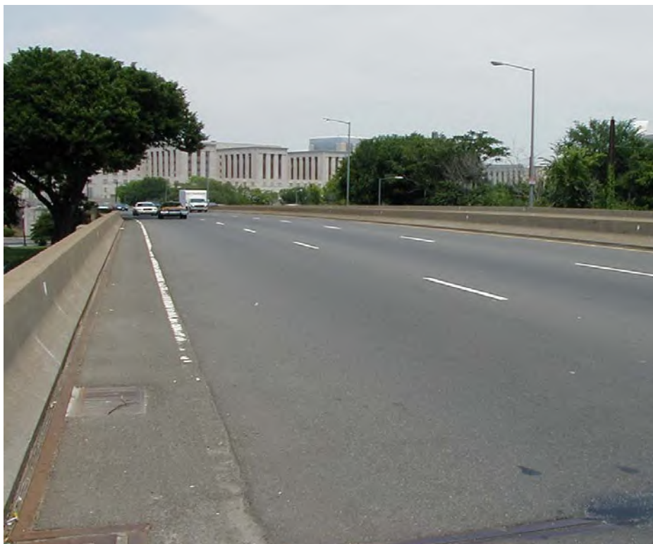
Figure 3.1.36 Asphalt Wearing Surface on a Concrete Deck
