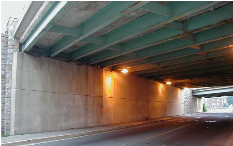
Figure 3.1.71 Cantilever Abutment (or Full Height Abutment)
