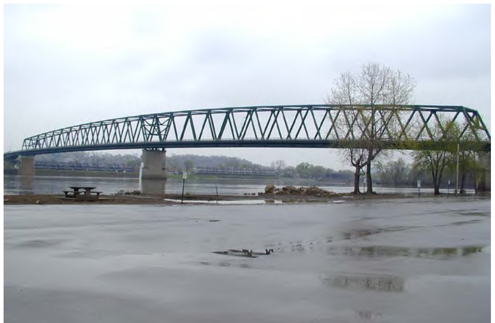
Figure 3.1.53 Through Truss Bridge
