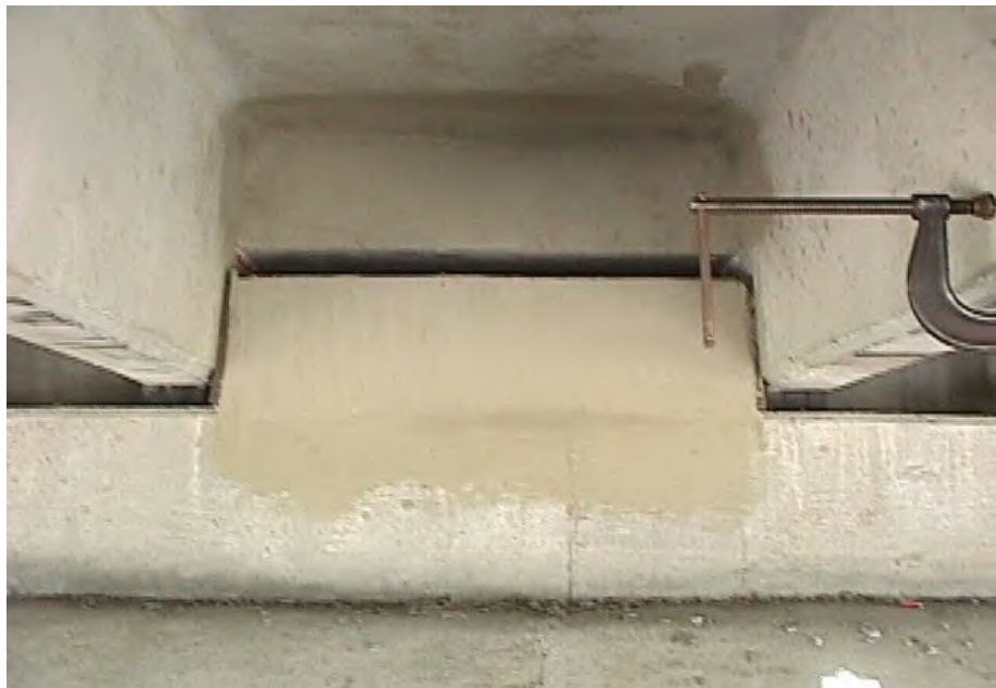
Figure 3.1.49 Tee Beam Bridge
